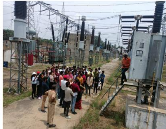
Industrial Visit to KPTCL Substation, Nelamangala Bengaluru Rural.
